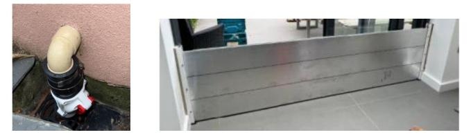
Above photos show an example of the works undertaken by our contractor. On the left is a non-return valve fitted to a waste pipe to prevent water backing up into the property. On the right is an aluminium slot in flood barrier to prevent surface water and fluvial (river) flows entering the rear of a property.
